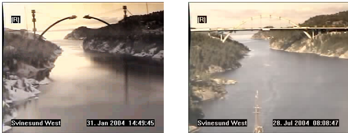
Figure 3: The Svinesund Bridge during construction
